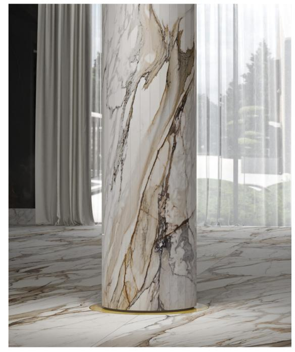
CUT-TO-SIZE VEIN MATCHING STRIPS FOR CIRCULAR COLUMN (FIG. 11.2)
