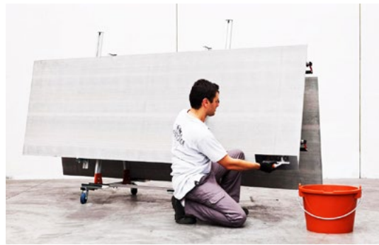
Back-buttering on transport cart
