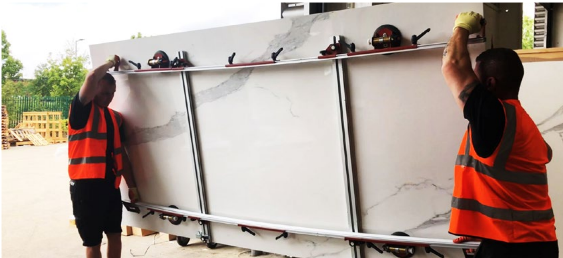
Always use handling frame to manoeuvre slabs
